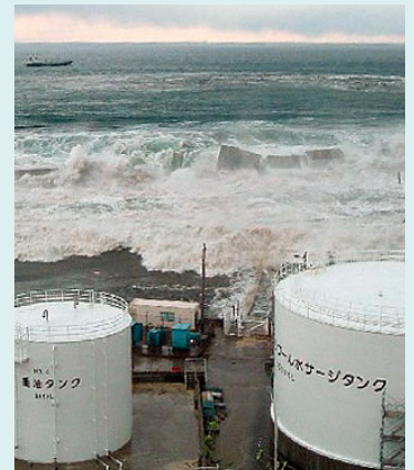
A major earthquake, followed by an exceptional tsunami, led to the failure or loss of all the emergency systems.
